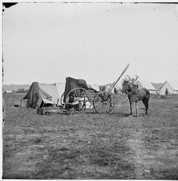
15 Civil War photo tent and wagon necessary for making light-sensitive plates in the field.
